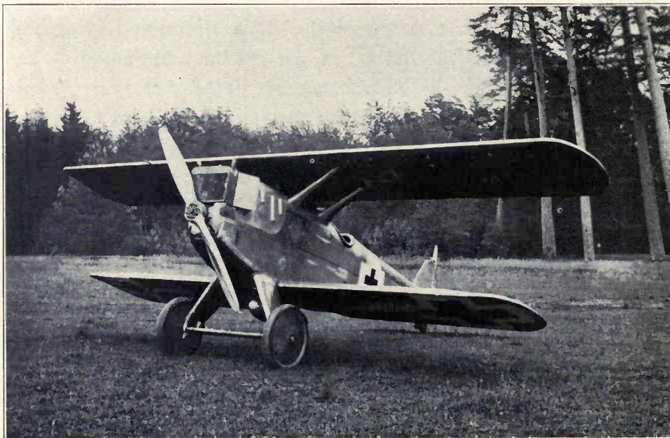
Zeppelin-Dornier All Metal Pursuit Plane Type DO D1, 1918. Note the absence of all struts and wire bracing.
